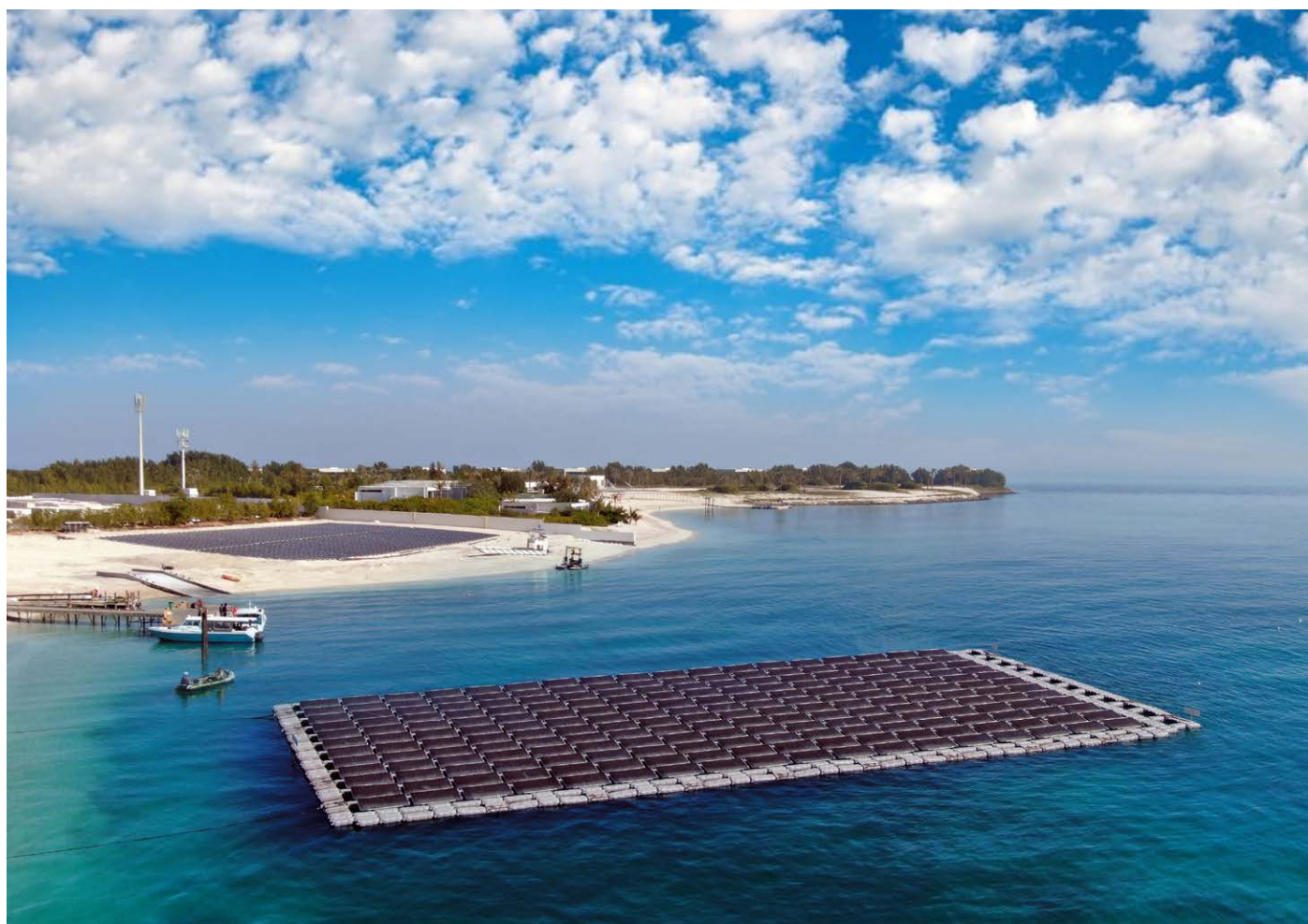
Middle-East near-shore 80kWp FPV Project (Courtesy of Sungrow Floating)
